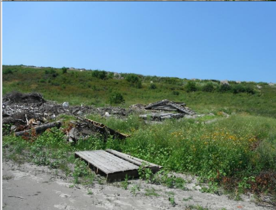
Photo 20: On access road looking west at the disturbed area at the toe of the landfill
