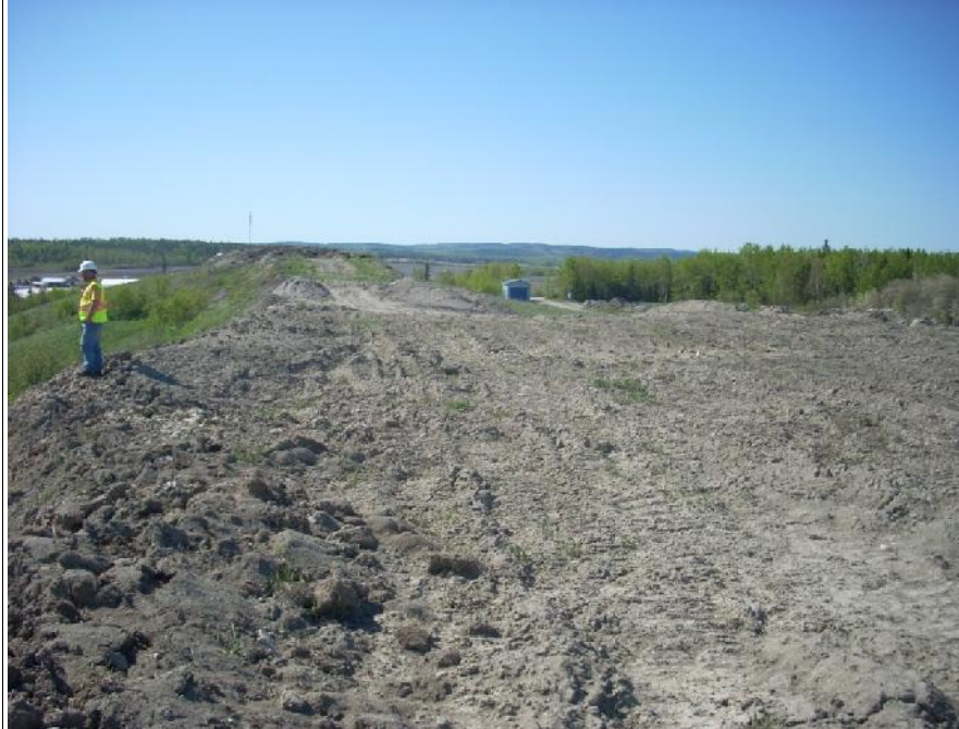
Photo 7: On top of existing landfill looking south towards gate entrance
