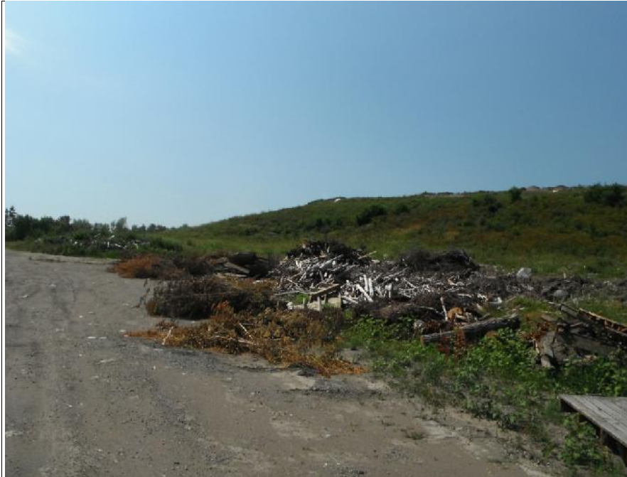
Photo 21: On access road looking southwest at the disturbed area at the toe of the landfill
