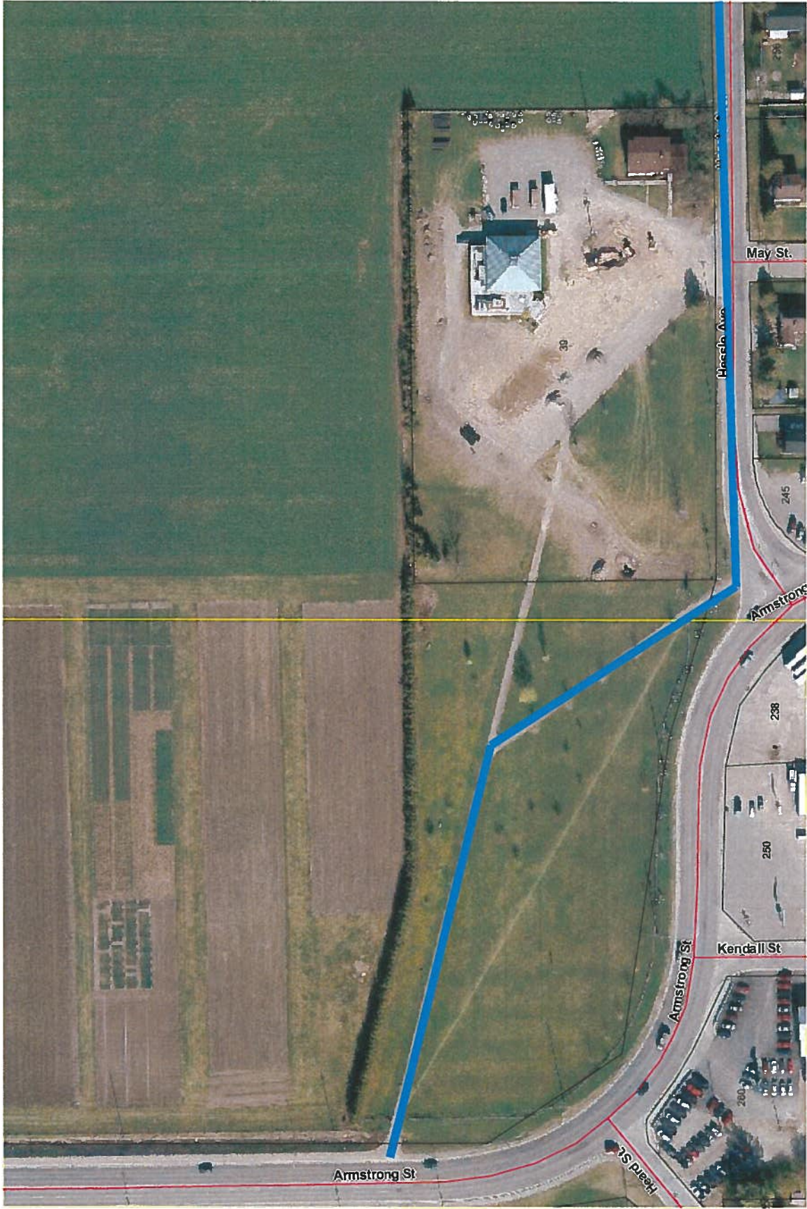
ARIO Property – Hesse Ave to Armstrong Street (2.5 metres width constructed / paved lane) 260m
