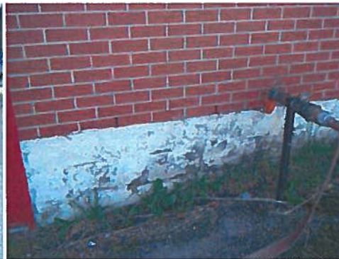
A42 – Foundation / Tanker Filler
