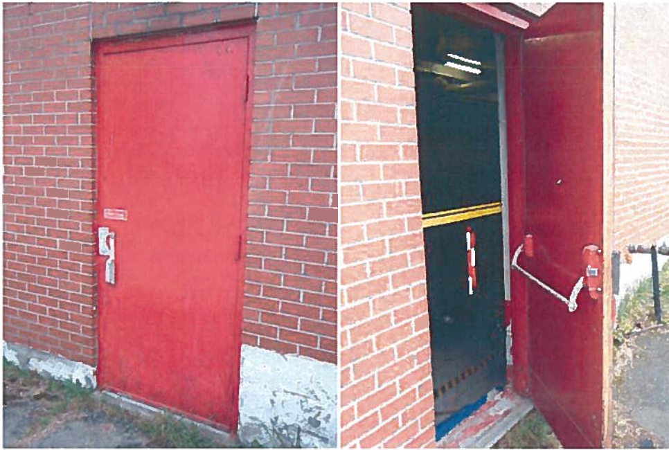
A43 & A44 – Exit Door North Face
