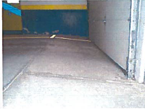
A38 – Sloped Floor Slab at O/H Doors
