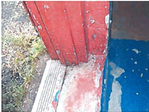
A45 – Exit Door North Face Sill
