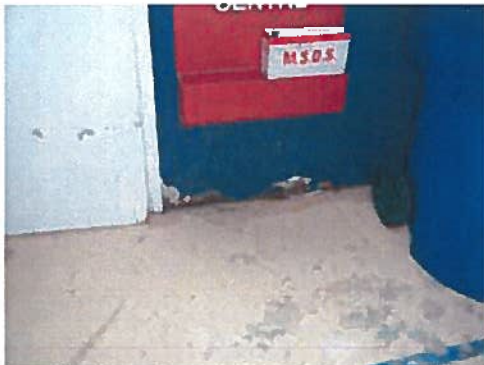
A19 – Water Damaged Drywall
