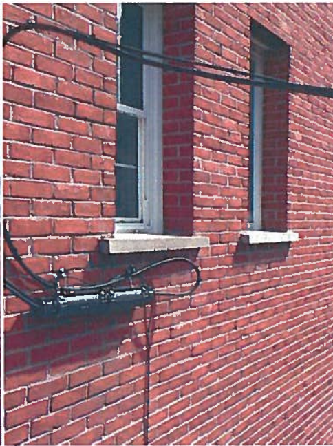
A48 – West Face 2 nd Floor Windows
