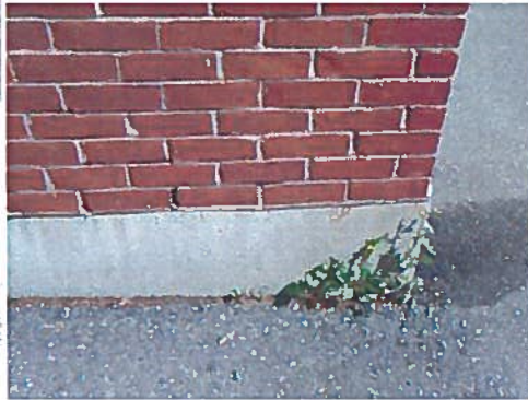
A57 – New Brick Veneer Junction w/ Existing A58 – Typical Parging on West face
