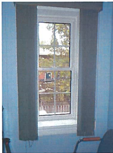
A74 – Typical Window in Chief's Office
