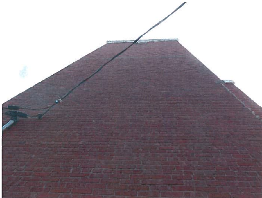
Figure 16: Typical masonry condition on the north face including hose-drying tower.
