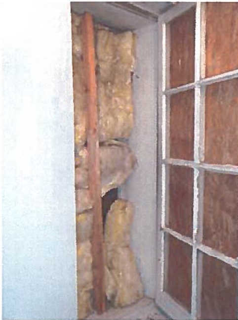
A77 – Original Window in Washroom Providing Access to Attic of Addition
