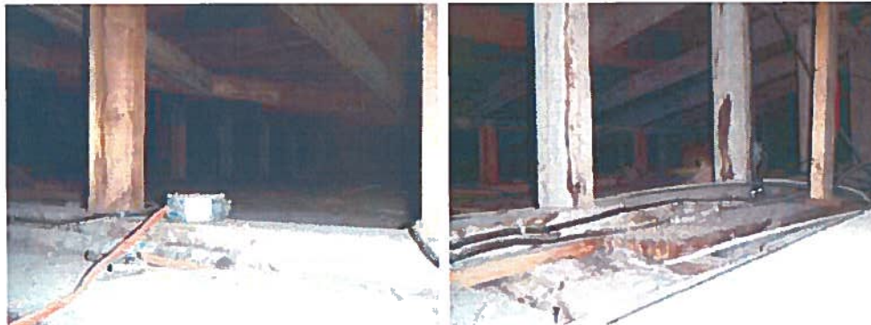
A81 & A82 – View of Original Hopped Roof Attic
