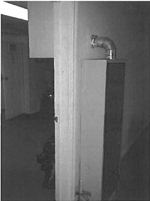
A67 – Gas Fired Unit Heater in Training Rm.
