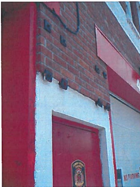
A31 - East Entry Door
