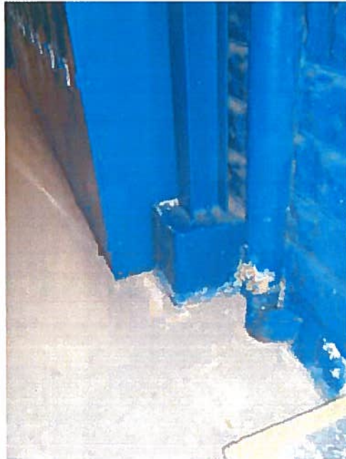
A30 – Base of Column (typical) – Addition
