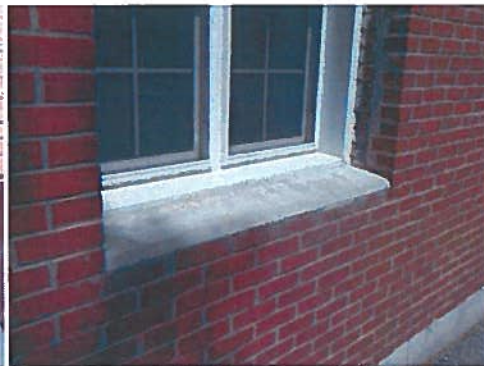
A50 – Parged Sill West Face Lower Floor
