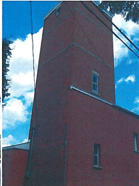
A4 - South Elevation (tower)
