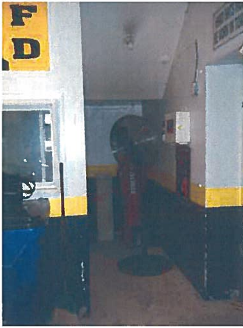
A25 - Hall to Former Basement Access Stair
