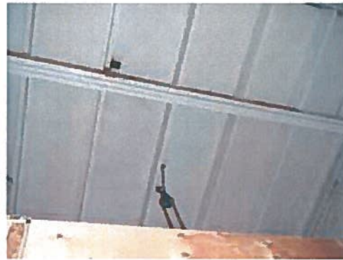
A46 – Hose Hoist Suspension at Ceiling
