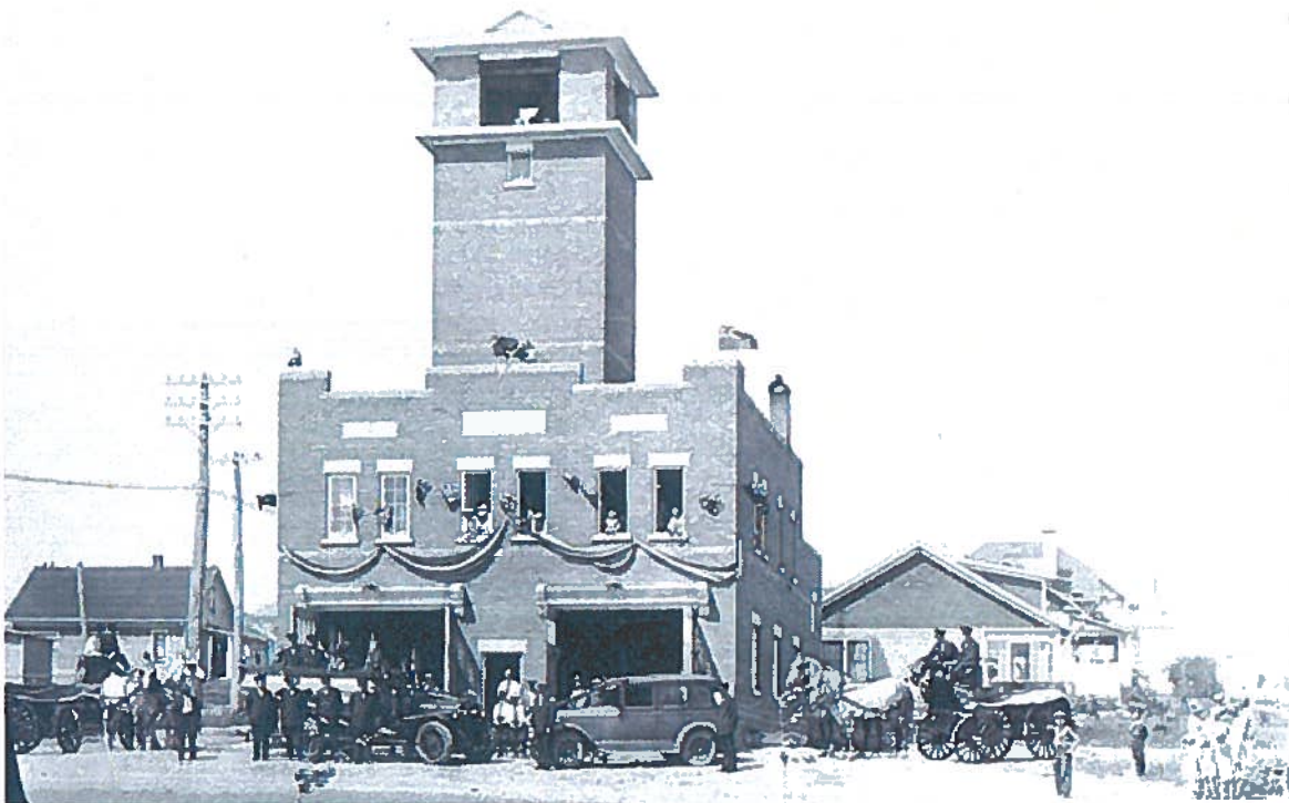
Figure 1: East face and northeast corner of the Haileybury Fire Hall circa 1923.
