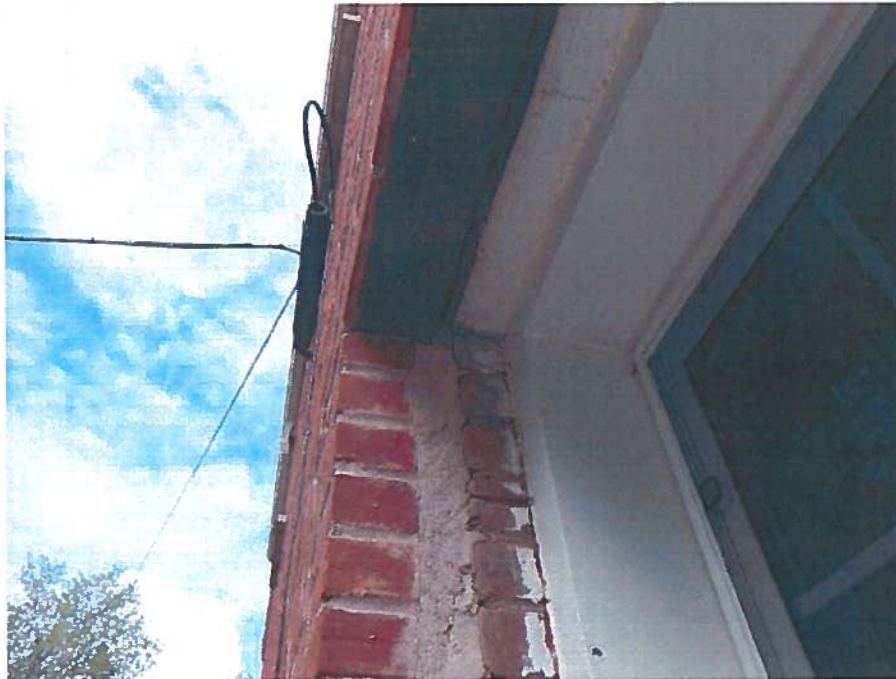
Figure 22: Typical detail around windows on the south face with newer masonry veneer.
