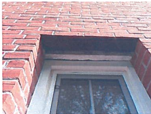
A49 – Open 'Soffit' West Face Windows
