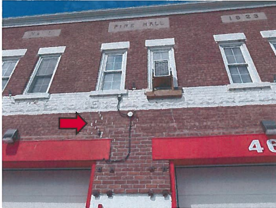
Figure 19: East face of 1923 building. Note evidence of previous crack repair.
