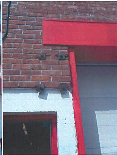
A32 - Typ. O/H Door Operator Thru Bolts
