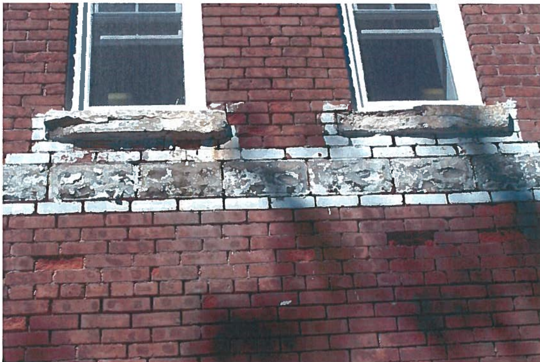
Figure 20: Condition of brick masonry on the south wall circa 2000 (prior to construction of new veneer).
