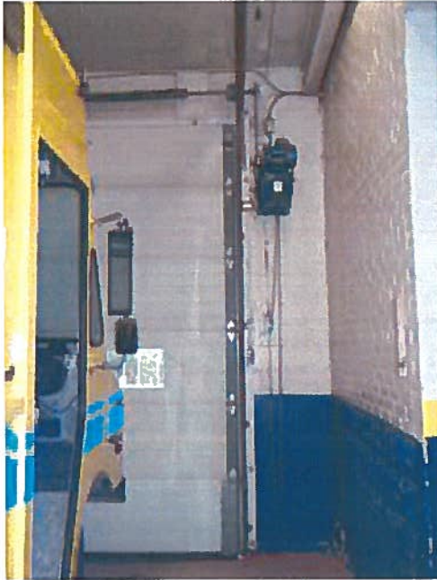
A7 – South East Corner - Addition
