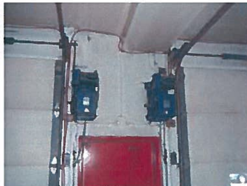
A18 – O/H Door Operators – Original Building
