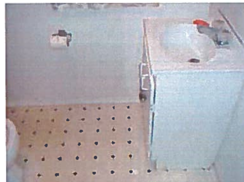
A65 – Second Floor Washroom Vanity
