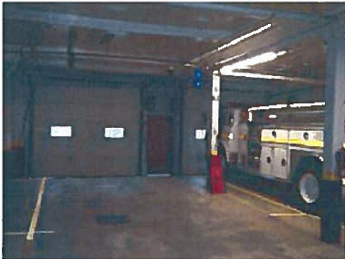
A1 & A2 – East Wall / Ceiling – Original Building
