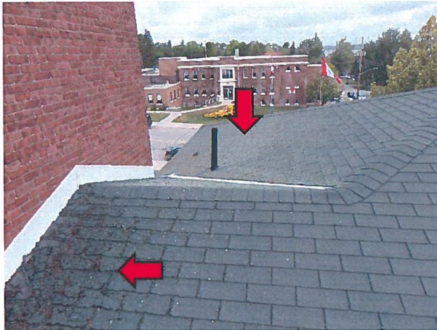
Figure 6: West half of roof. Note shingle deterioration and moss/lichen growth beyond.
