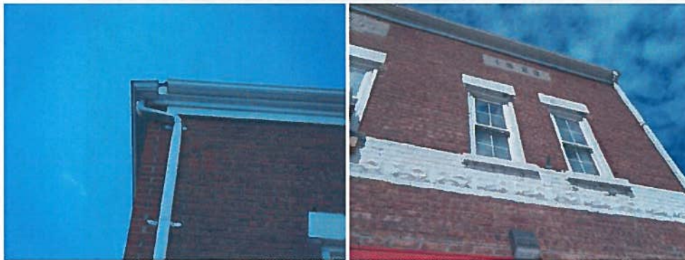
A29 – East Face, South End Eavestrough
