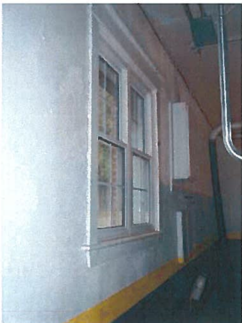
A5 – South Wall – Original Building
