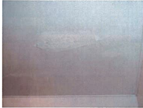
A76 – Delaminating Ceiling in Storage Room
