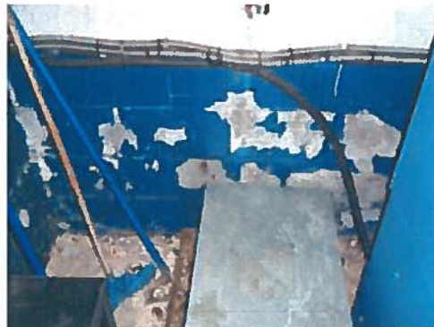
A20 – Below Grade Paint Peeling – West Wall
