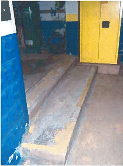
A33 – Typical Steps Down to Addition
