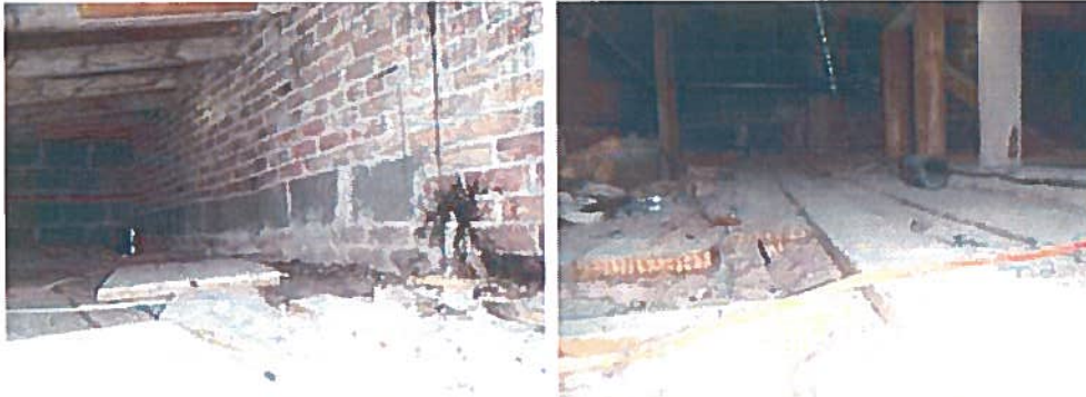
A79 & A80 – View of Original Hopped Roof Attic (Tower wall in Background)
