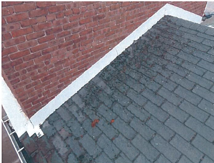
Figure 8: Advanced shingle deterioration east of hose-drying tower.
