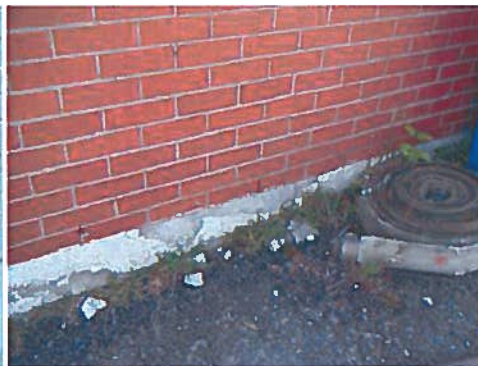
A40 – Parging Damage - Addition North Face
