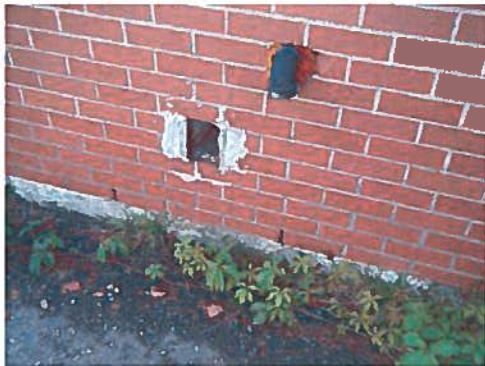
A53 – Rough Brick Patching North Face
