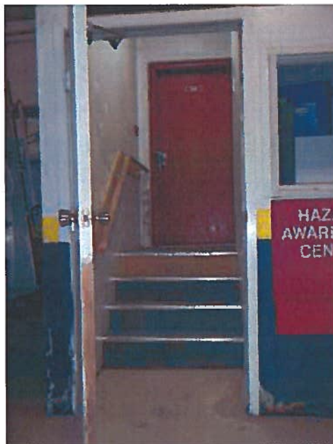
A23 – Stair Entry to Vehicle Bays
