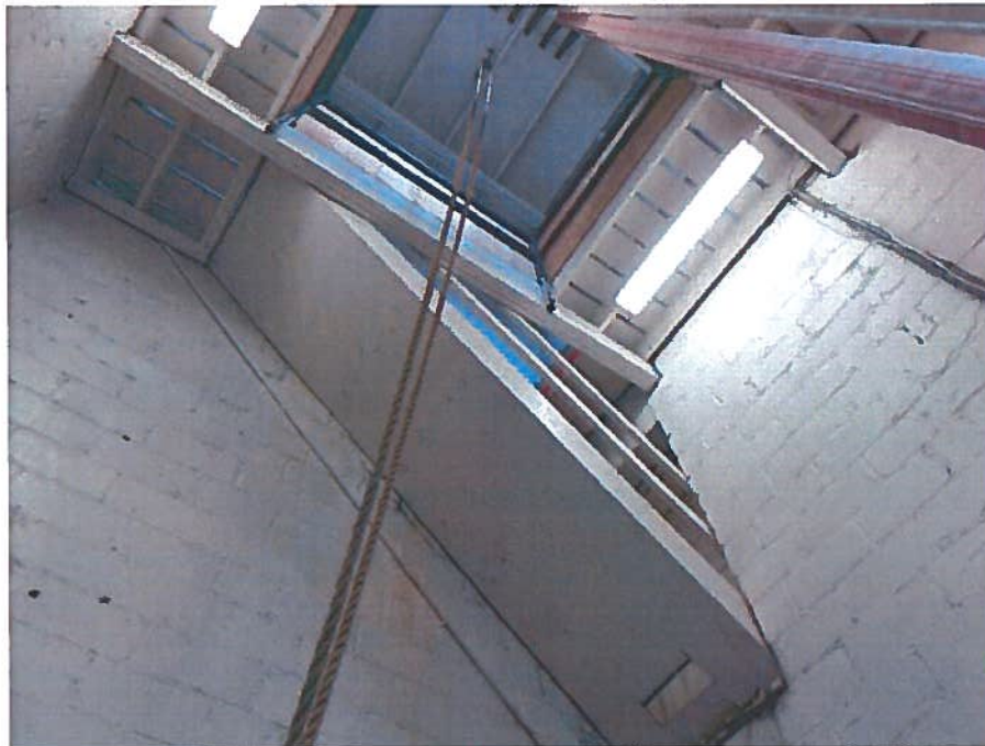
Figure 14: Hose-drying tower platform framing and access stair.
