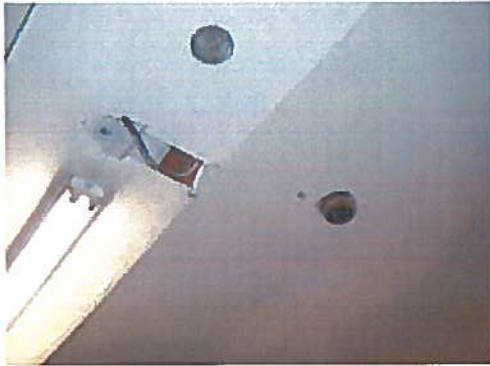
A37 – Fire Rating Breach Vehicle Bays
