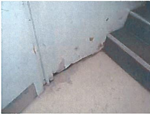
A53 – Wall Damage at Bottom of Stair
