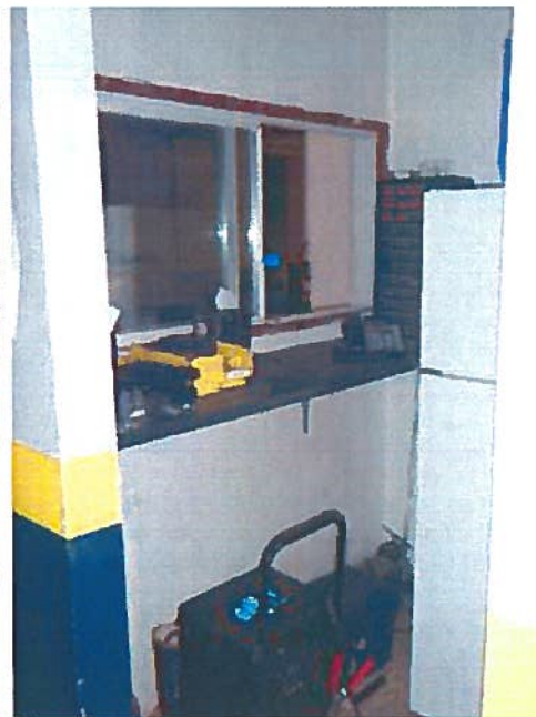
A24 – Inside Former Dispatch Office
