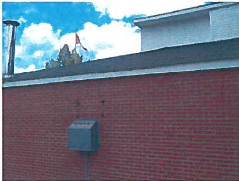
A15 – Low Roof Shingles, West Side
