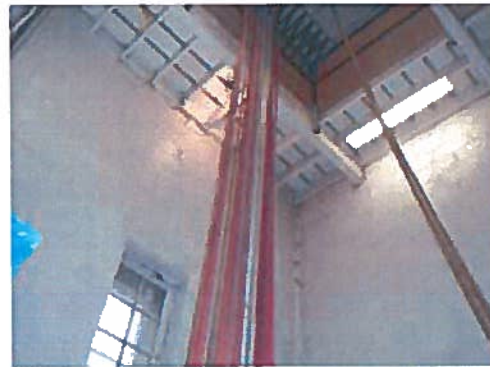
A41 & A42 – Interior Views of Hose Tower
