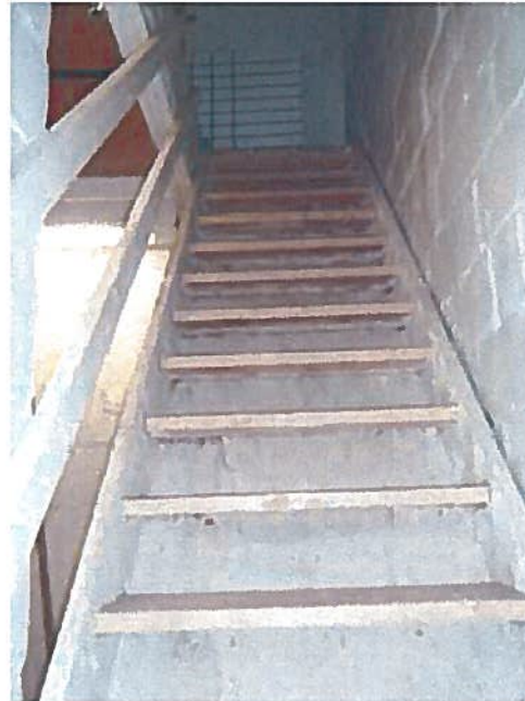
A48 – Wood Stair up to Top of Hose Tower
