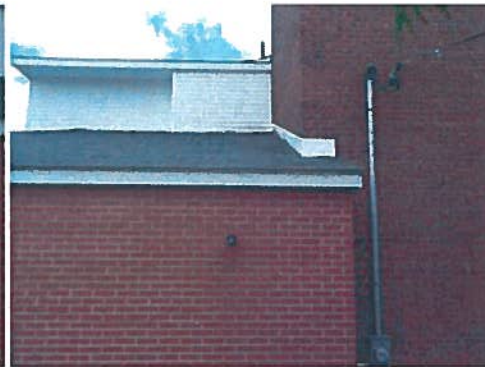
A16 – Low Roof Shingles, West Side
