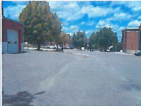
A2 – East Driveway Looking North
