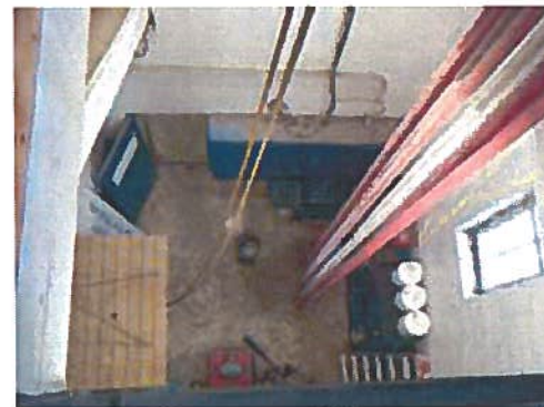
A43 – Interior View of Hose Tower
