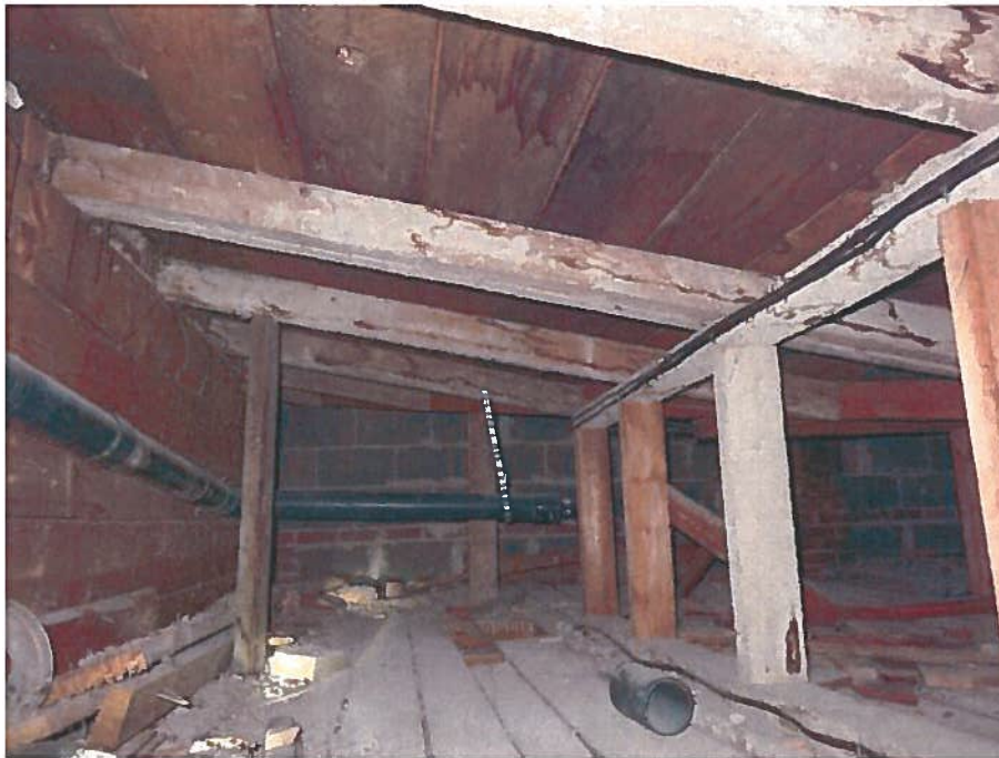
Figure 4: Attic above 1923 building looking north.
