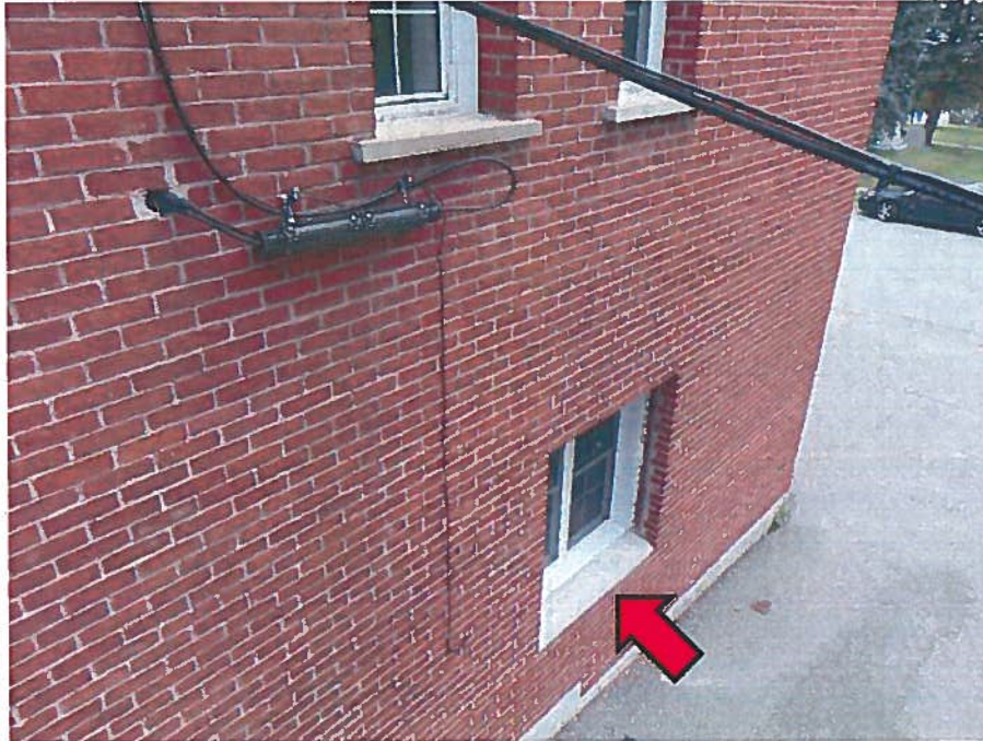
Figure 21: Southwest corner of the newer masonry veneer. Note window sill without drip edge.
