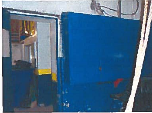
A39 – Elect. Panel Cabinet – Hose Tower
