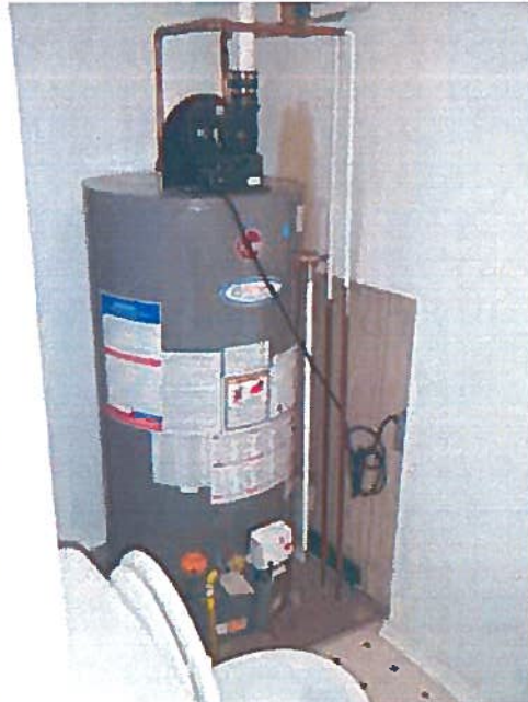
A64 – Gas Hot Water Tank in Washroom
