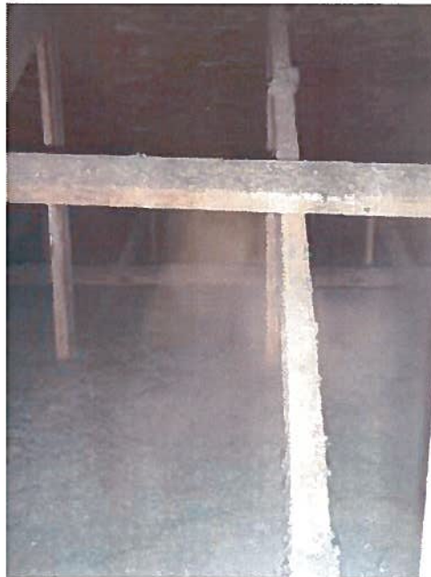
A78 – View of Attic Through Access 'Window'
