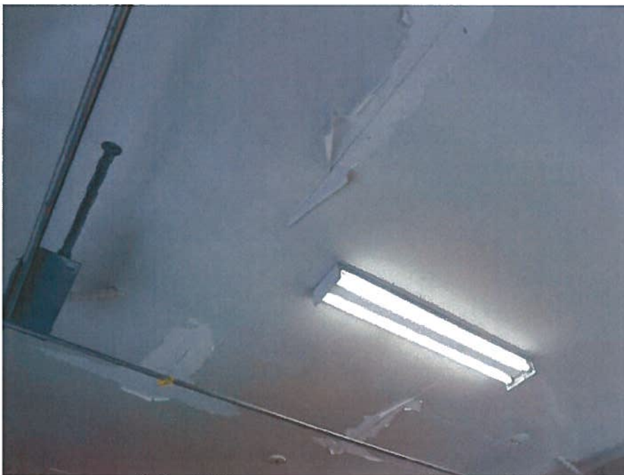
Figure 12: Cracking and peeling ceiling below south half of Second Floor.
