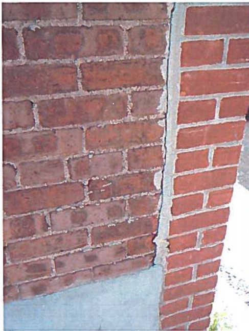
A57 – New Brick Veneer Junction w/ Existing A58 – Typical Parging on West face
