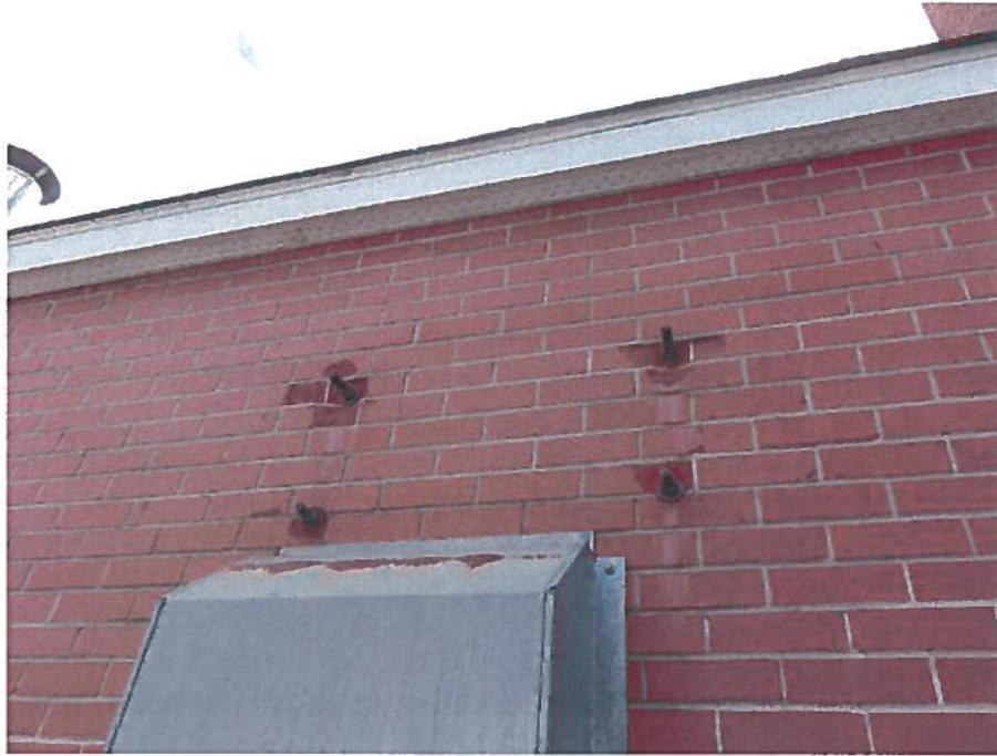
Figure 27: Corroding steel bolts and associated masonry damage on the west face of the 1971 building.
