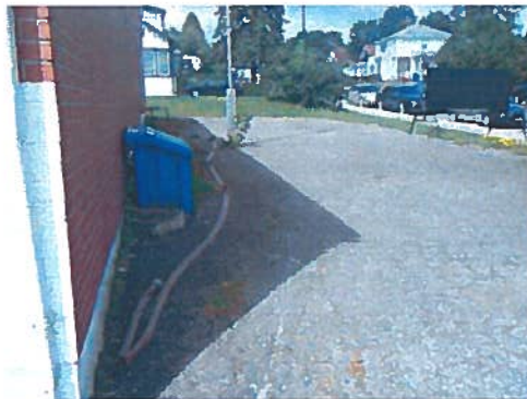
A41 – North Laneway Looking West
