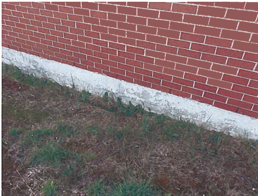
Figure 28: Typical condition of the foundation wall parging observed along the north face of the 1971 addition.
