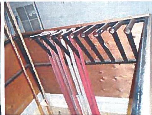
A44 – Hose Rack – Top of Hose Tower
