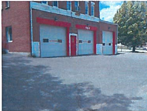
A21 – East Driveway
