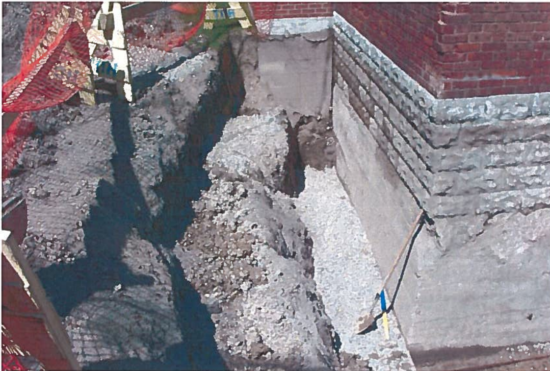
Figure 15: Exposed foundations at southwest corner of 1923 building circa 2000. Note 1971 foundations visible beyond.
