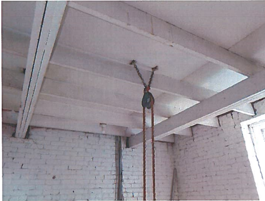
Figure 13: Hose-drying tower roof framing and hoist block.
