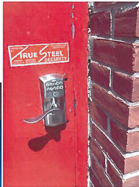
A46 – Door Hardware West Face
