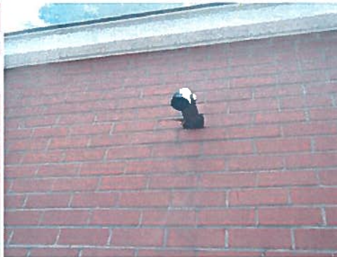
A54 – Unsealed Penetration West Face
