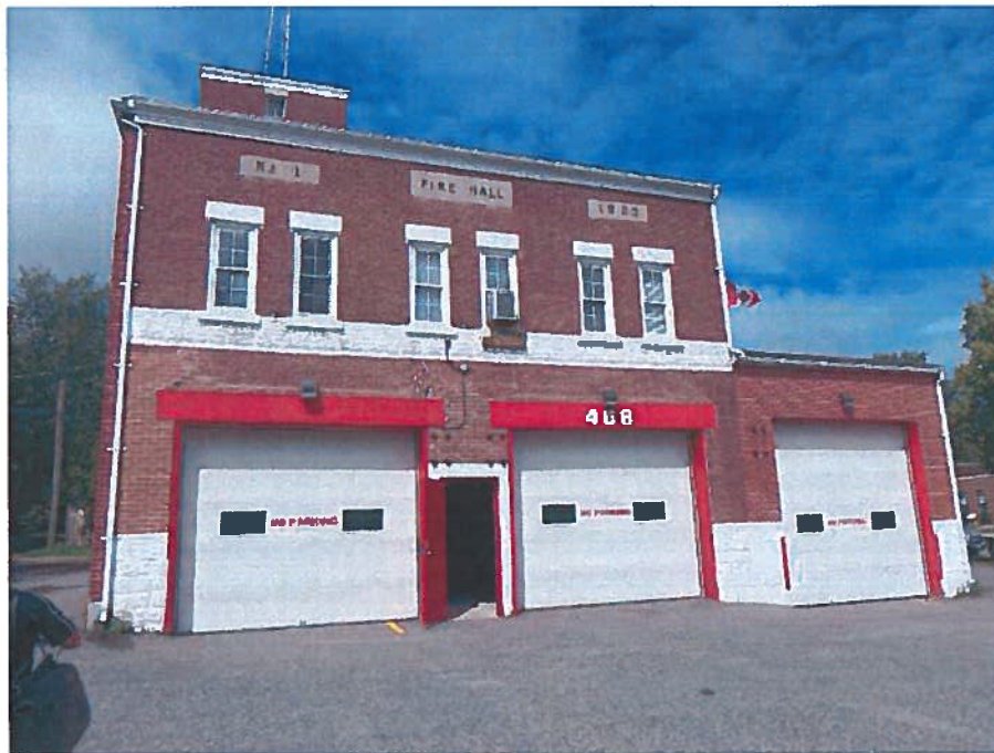
Figure 2: East face of the Haileybury Fire Hall circa 2015.
