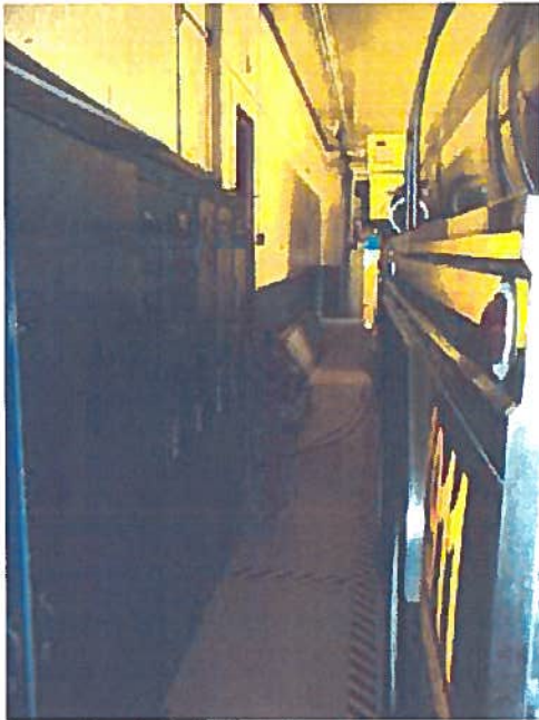
A21 – North Wall – Addition
