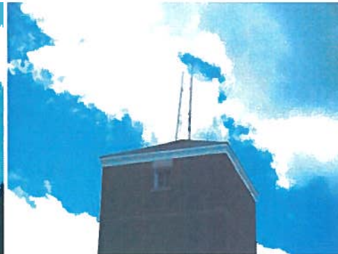
A18 – Tower Roof, South Side
