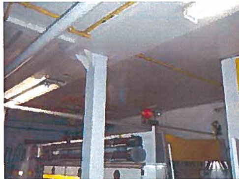
A9 & A10 – Ceiling of South Bay – Original Building
