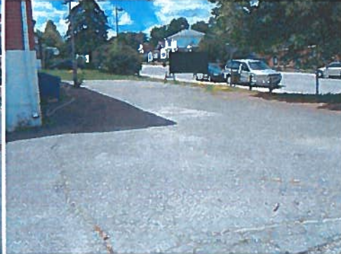
A24 – North Laneway Looking West
