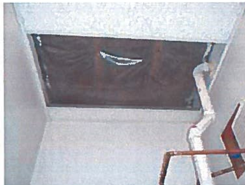
A66 – Washroom Ceiling / HWT Vent
