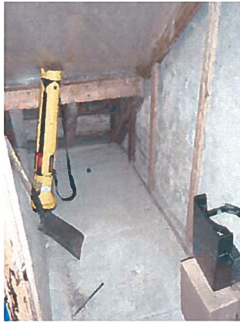
A26 - Concrete Filled Basement Access Stair
