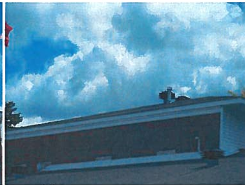
A14 – High & Low Roof Shingles, North Side
