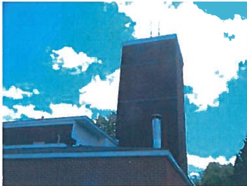
A17 – Tower & Roof at North West Corner
