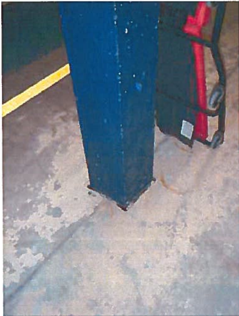
A29 – Base of Column – Original Building
