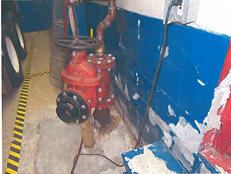
Figure 25: Evidence of water infiltration on north side of 1971 addition.
