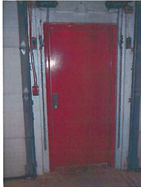
A32 – East Entrance Man Door
