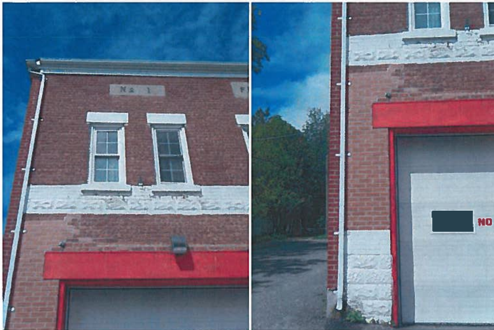
A27 & A28 – East Face, South End – Brick Cracking & Settlement / Previous Repair
