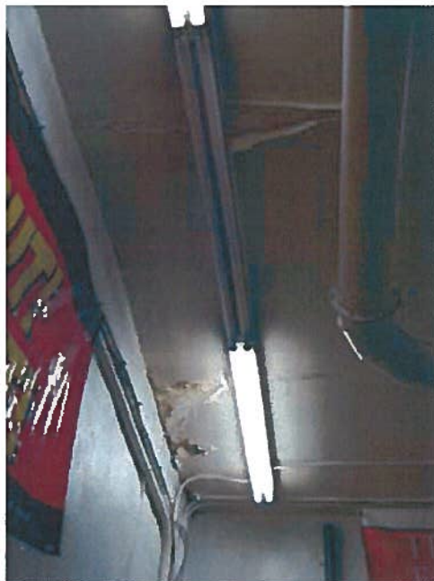
A36 – Water Damage / Paint Peeling Ceiling of Addition
