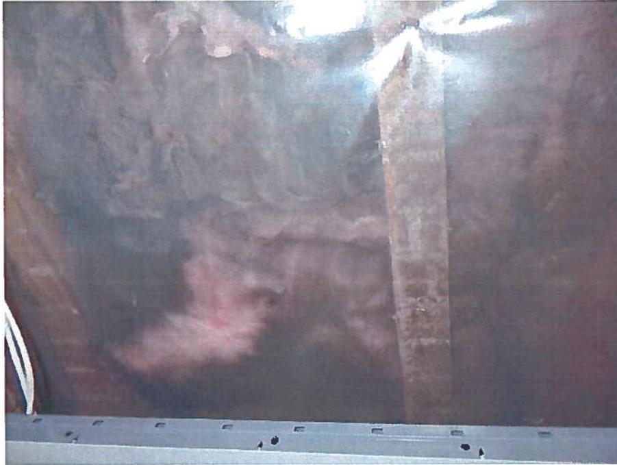
Figure 5: Exposed ceiling joists, insulation and vapour barrier in 1923 roof.
