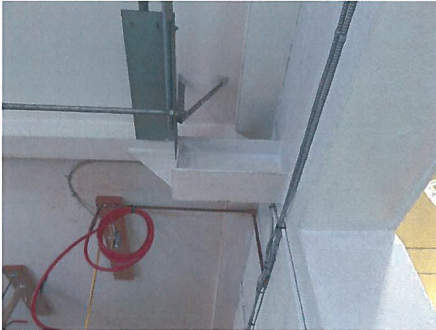
Figure 11: Steel beam extension beam below Second Floor.
