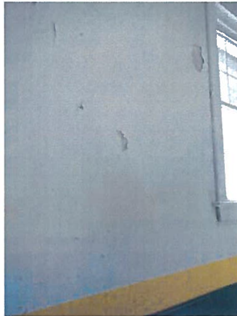
A28 - South Wall - Plaster Delamination
