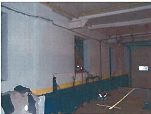
A3 & A4 – North Wall – Original Building
