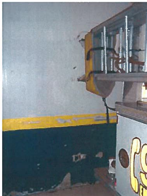
A6 – Rear Wall Damage – South Vehicle Bay
