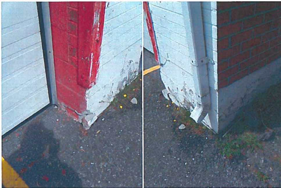
A37 & A38 – O/H Door / Foundation at Addition – North East Corner
