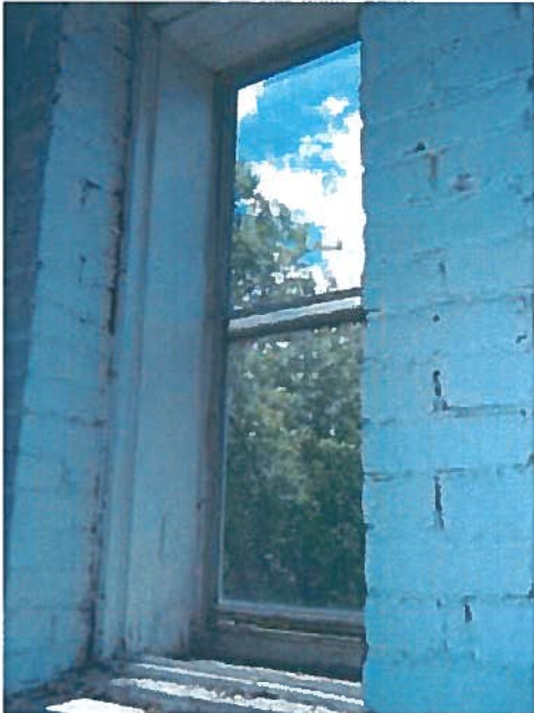
A47 – Original Window Inside Hose Tower
