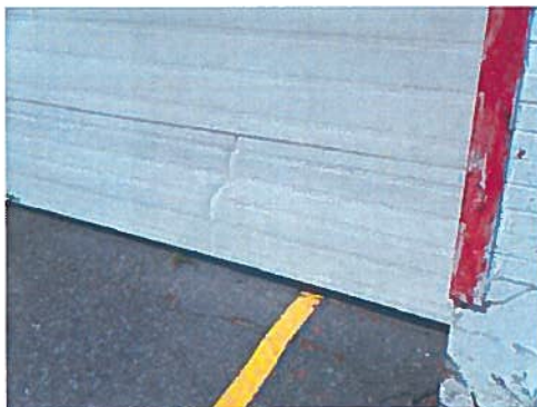
A39 – O/H Door Damage at Addition
