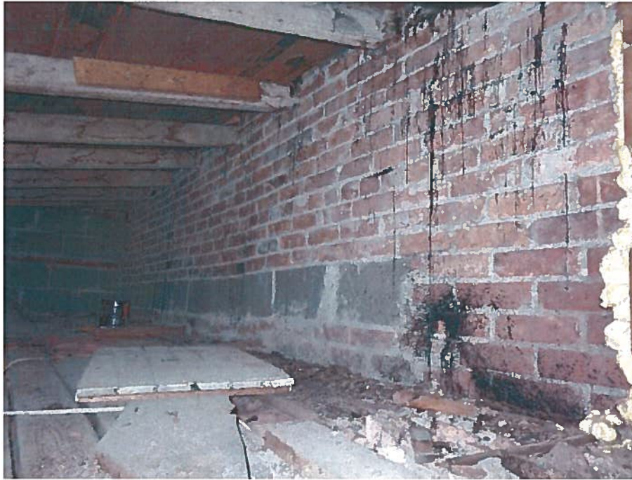
Figure 3: Attic above the 1923 building. East face of the hose-drying tower shown.
