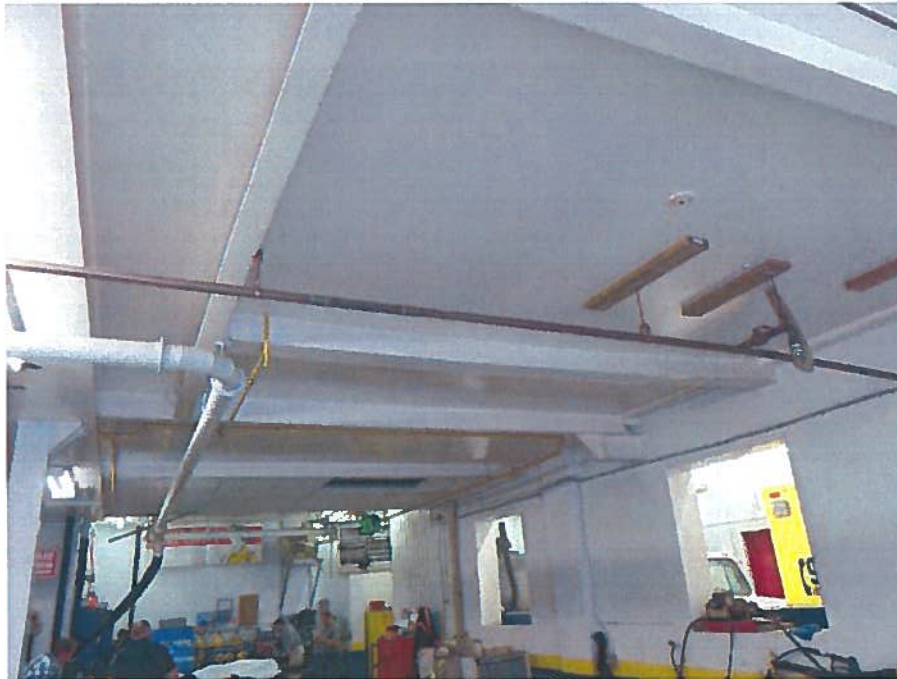
Figure 10: Beams below north half of Second Floor.
