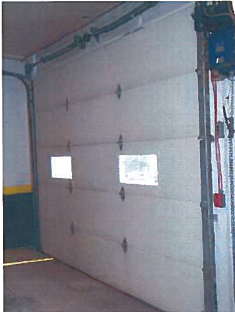
A31 – Overhead Door – Original Building
