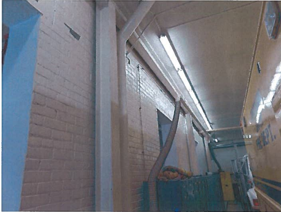
Figure 23: Structural steel framing associated with 1971 addition adjacent to the original north wall.
