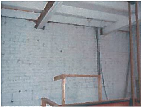
A45 – Hose Tower Ceiling / Wall Junction
