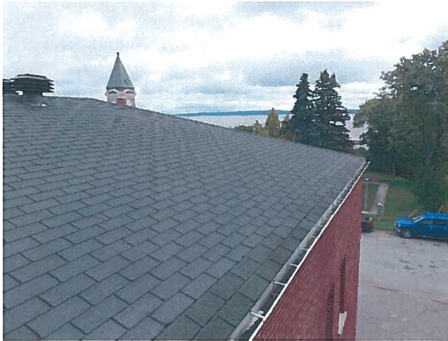
Figure 7: Southeast corner of roof on 1923 building.
