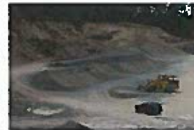
Loose material like sand & gravel is extracted from sites called "pits"
