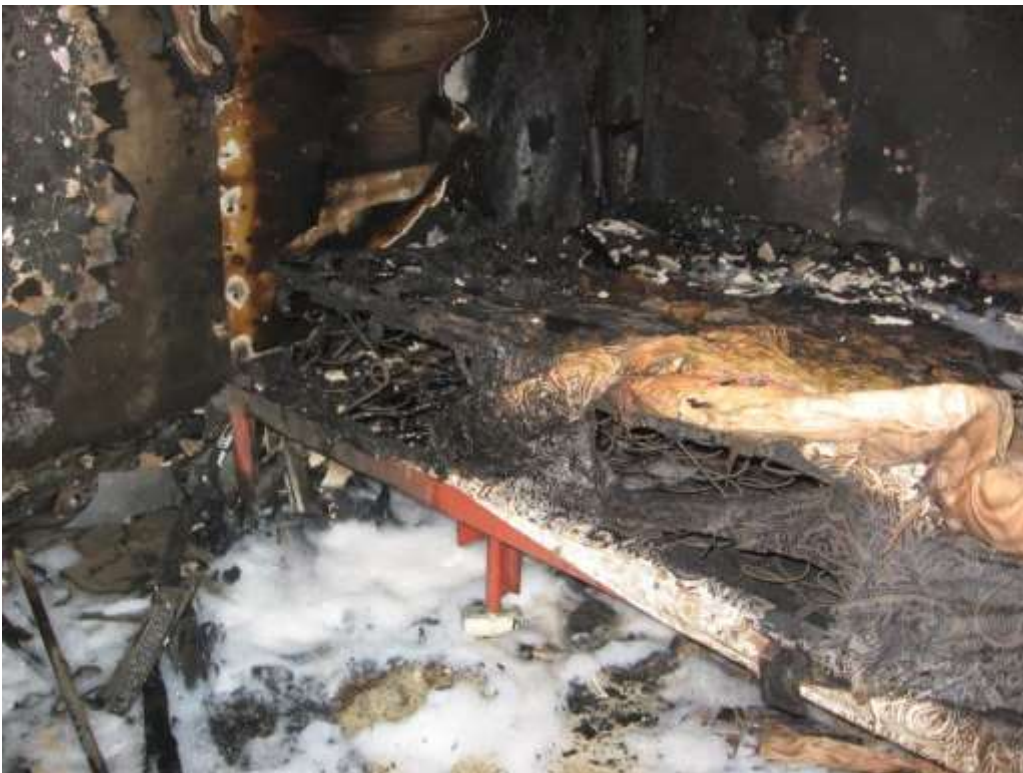
July 24, 2017 – Structure Fire, Kendall Street
