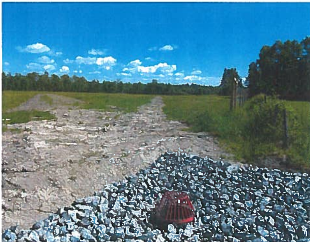
Drain Post Construction
