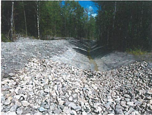
Erosion Control Measures
