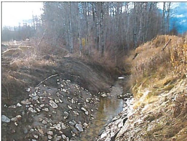
Drain Post Construction
