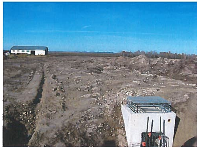
Drain During Construction
