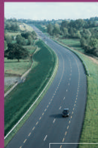
Typical wide two lane road
