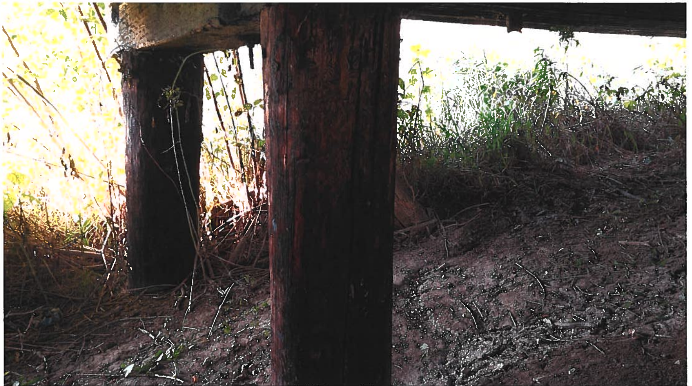
10. Split - First Pier from West, Second Pile from South
