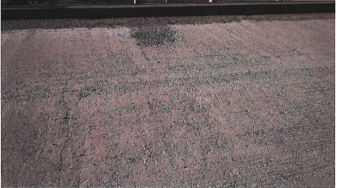
5. Deck - Transverse Cracks Throughout
