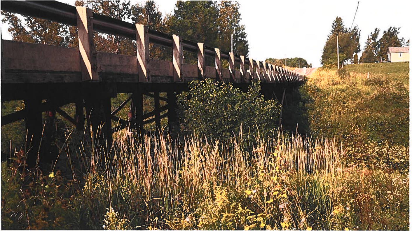
3. North Elevation (looking south)
