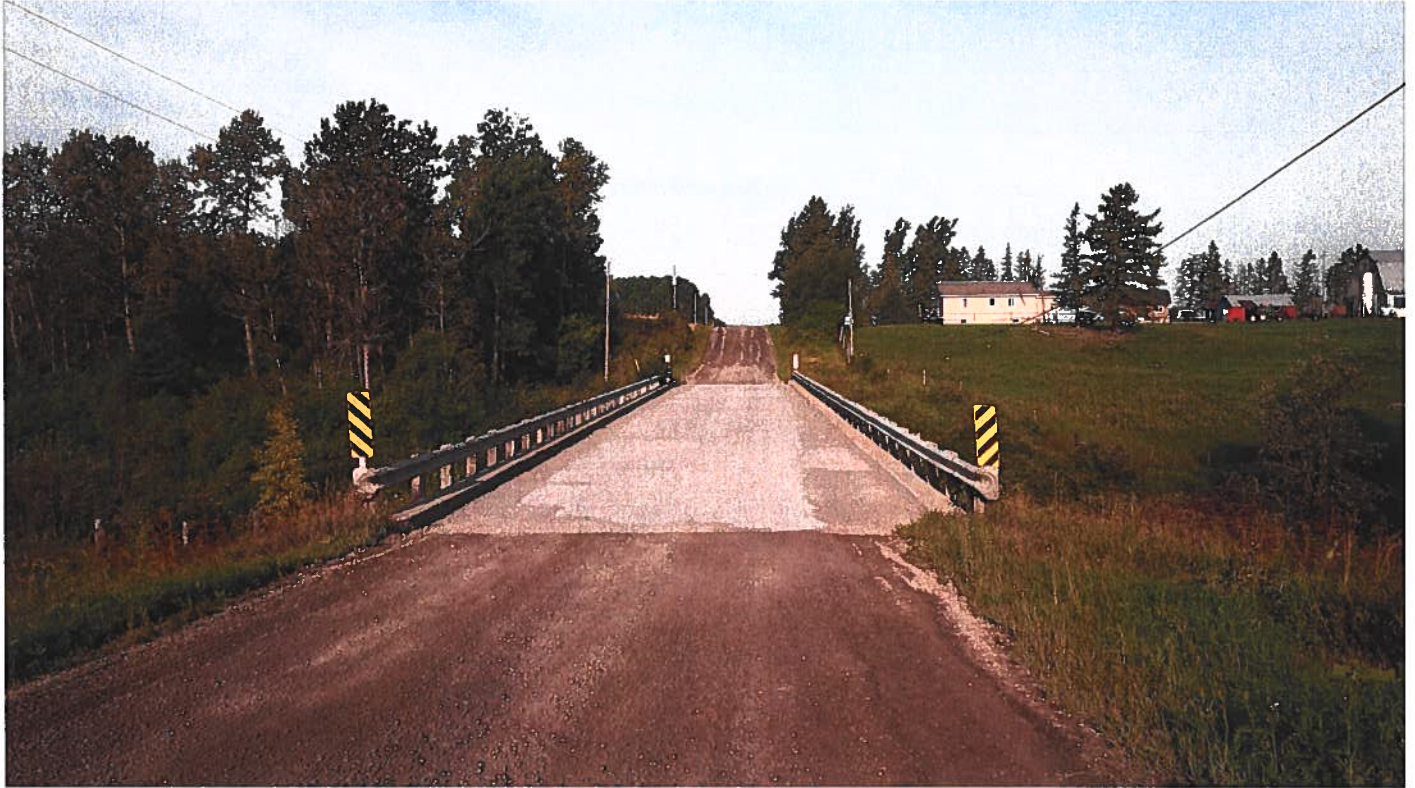
1. East Approach (looking west)
