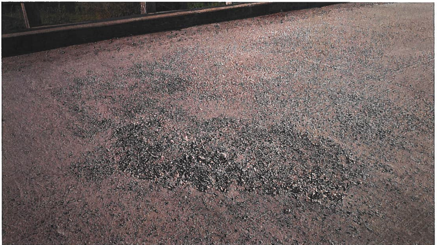
6. Deck - Severe Scaling
