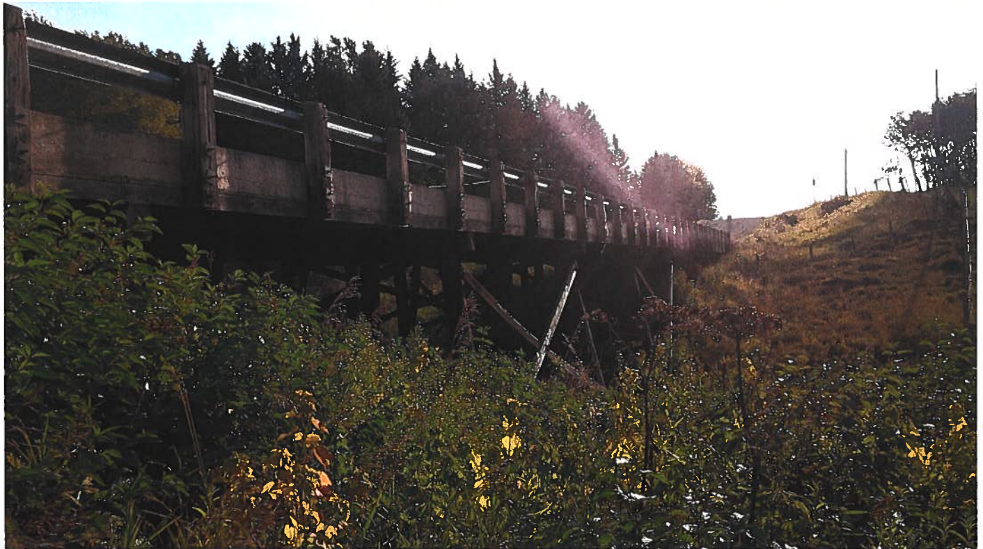
4. South Elevation (looking north)
