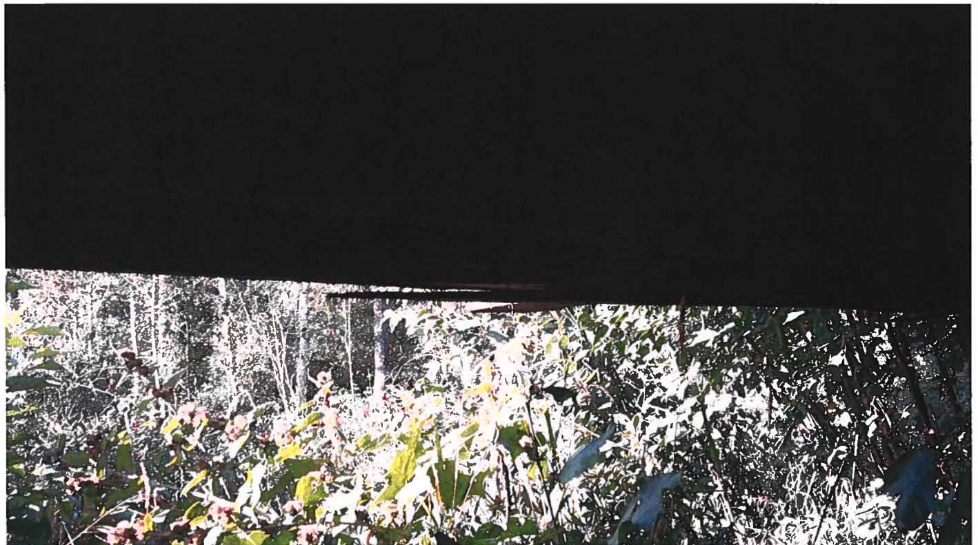
12. Deck - Splinter at Southwest
