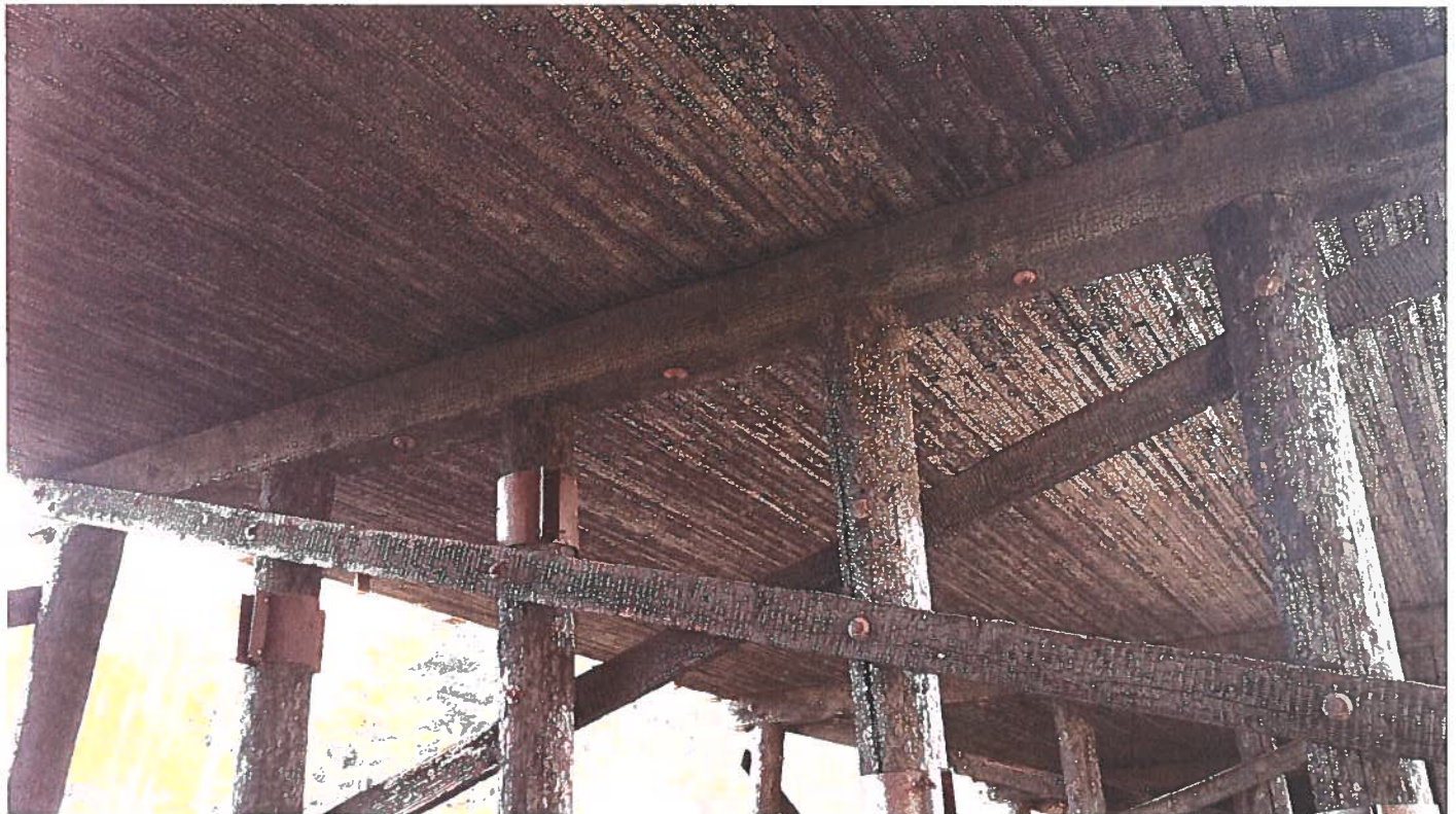
8. Soffit - Fire Damage
