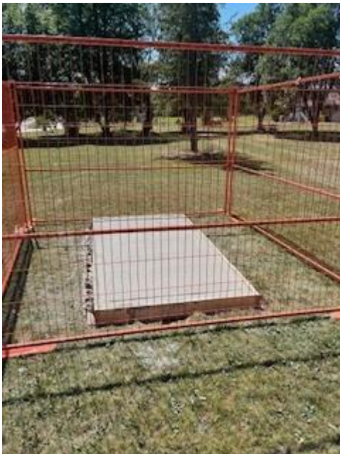
Figure 3 – A recently completed concrete pad for a memorial bench installation
