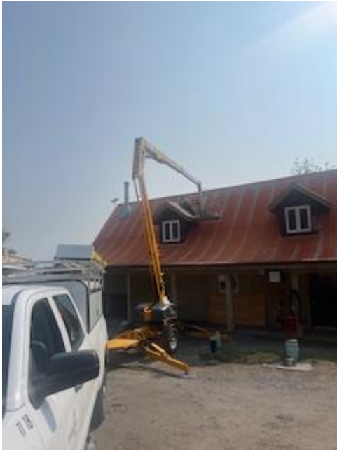
Figure 1 - City staff repair the roof of the Chalet at Bucke Park
