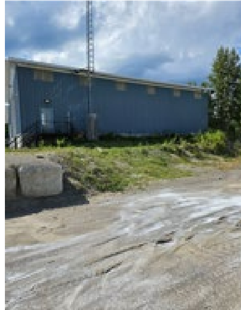
Figure 2 - City staff removed vegetation which had been left to grow next to various buildings for multiple years.
