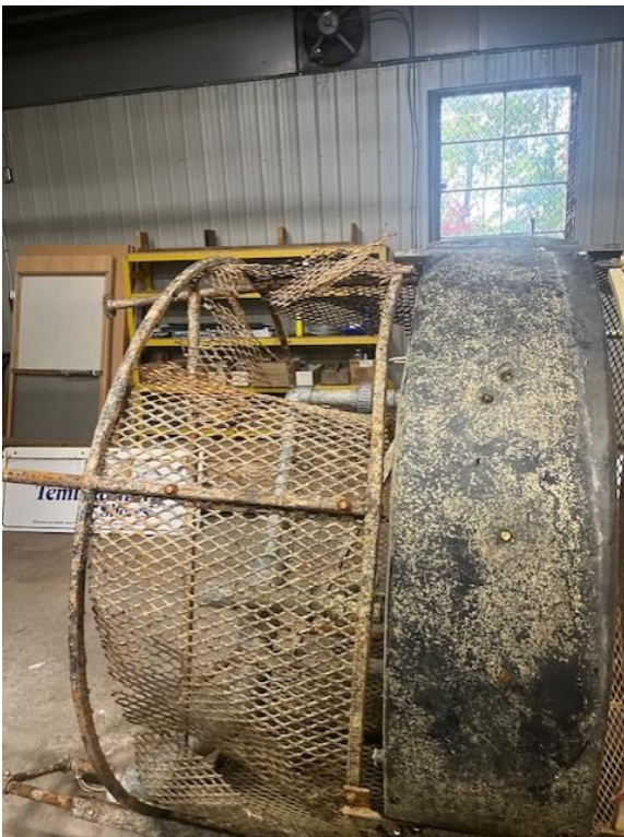
Figure 3 – Damage on the Haileybury Beach fountain which will need to be repaired over winter. The issue appears to stem from some broken floats.
