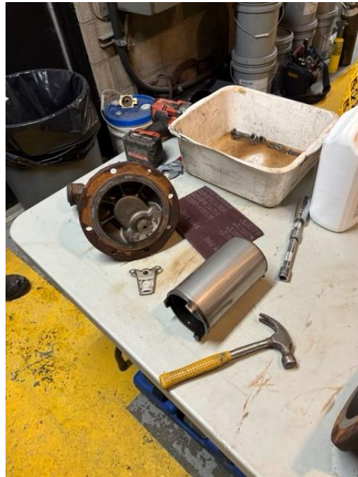
Figure 2 - The high-side float for the DSMA ice plant needed to be disassembled and replaced.
