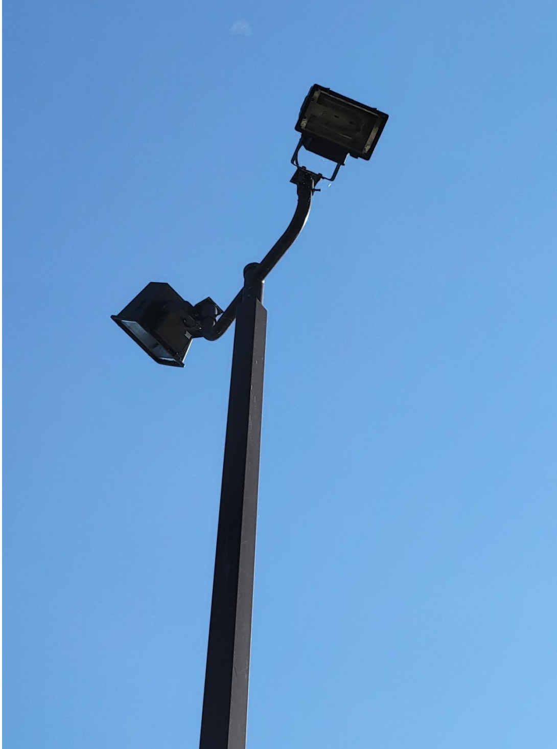
Figure 2 - Existing Double Fixture Pole
