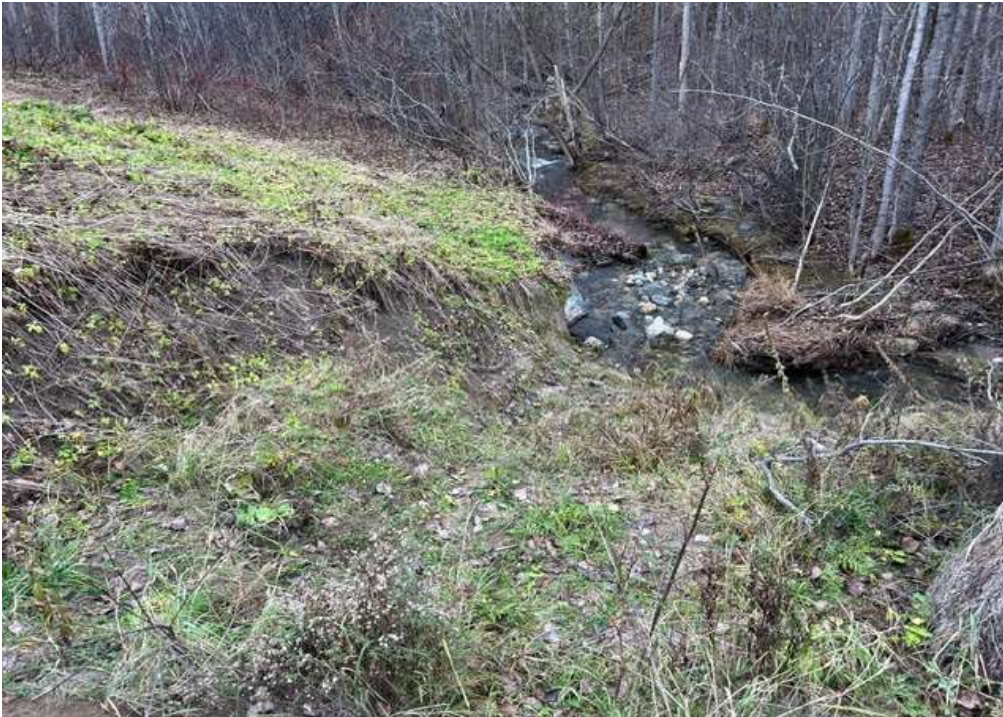
Photo #3 - The toe of the slope.
